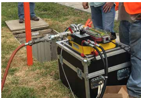
Outdoor Microduct optical fiber cable installation by blowing
