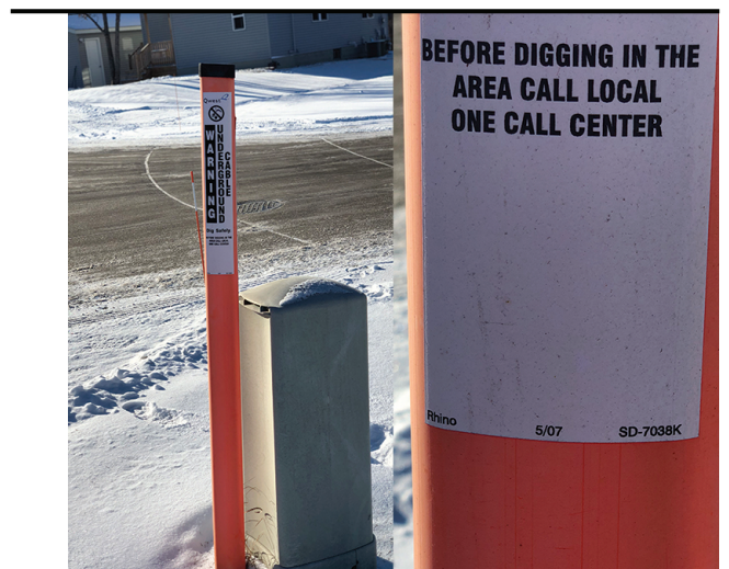
Photo taken 4/2018 • TriView install date 5/2007
