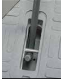
Recessed Lifting Pin with Cover
