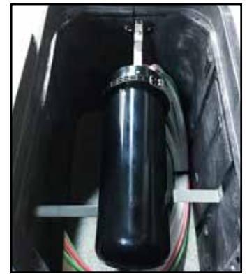
90° Splice closure mounting
